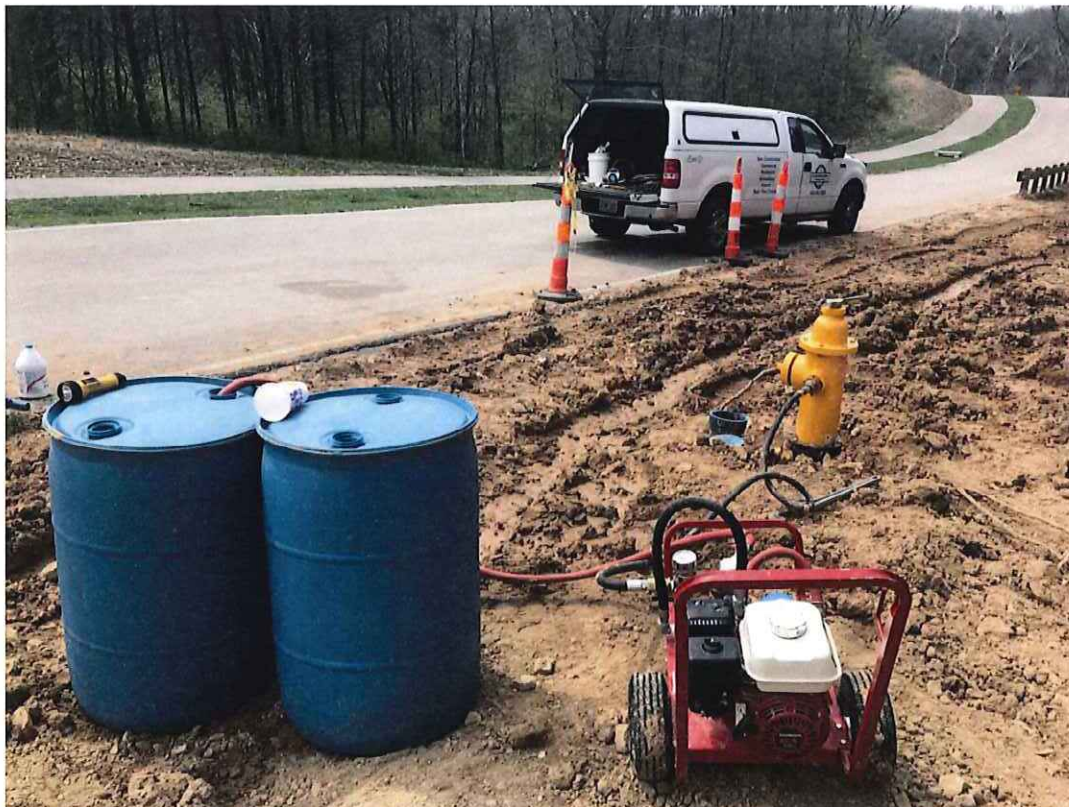
Photo 1 – Tools to test the water line for any leaks.
