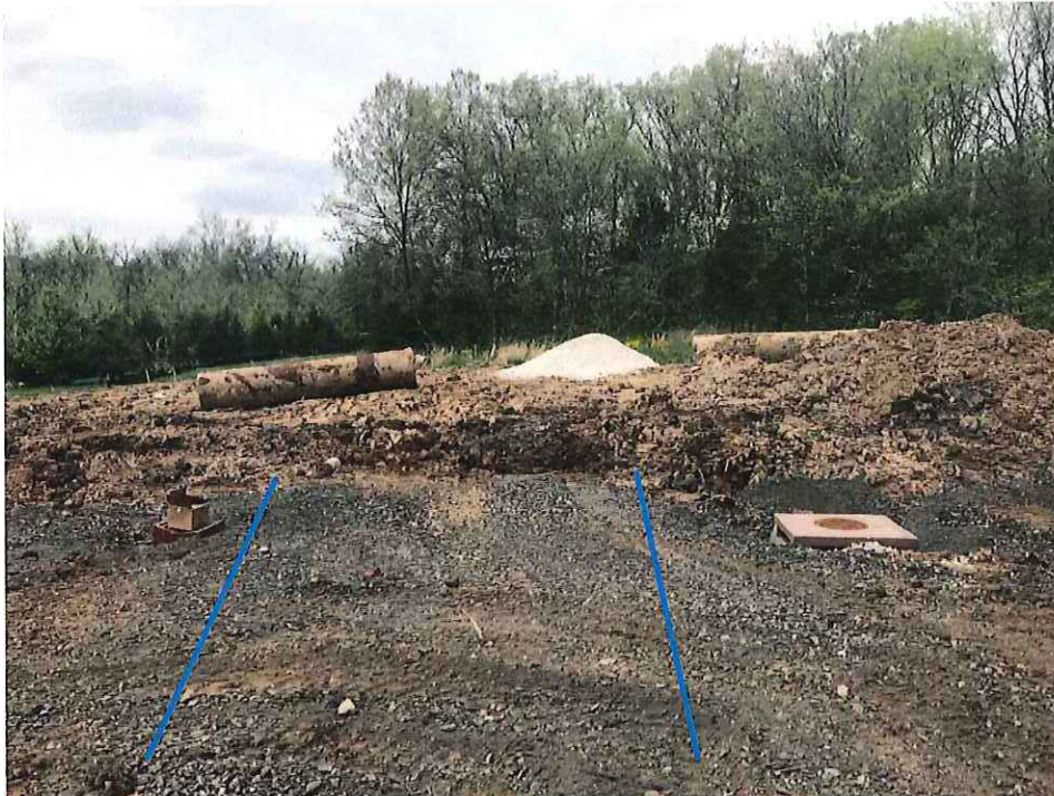
Photo 1 – New pipe crossing under the proposed Access Road.
