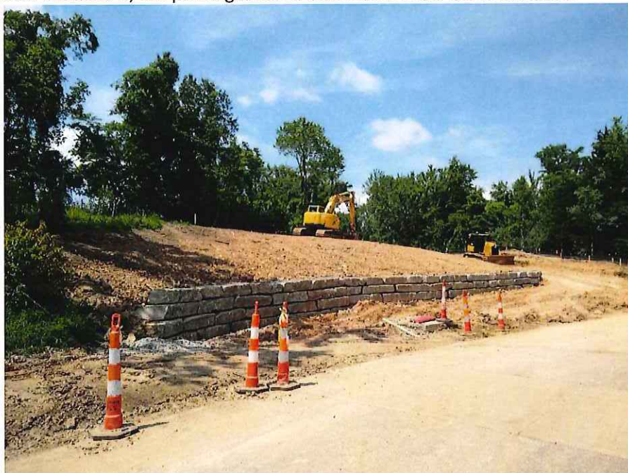
Photo 1 - Looking at retaining wall from Park Drive.
