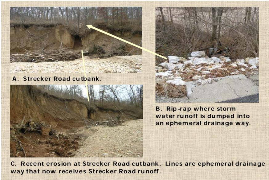
Figure 1. Three (3) views of Strecker Road cutbank. “A” is from the stream toward Strecker Road. “B” is from Strecker Road toward Caulks Creek, looking down toward the rip-rap below the new storm water runoff pipe that dumps into the creek. “C” is a view along the cutbank showing recent erosion. The arrow from B to A shows the rip-rap in Figure A. The line in A and C shows the same ephemeral drainage way in both photographs.
