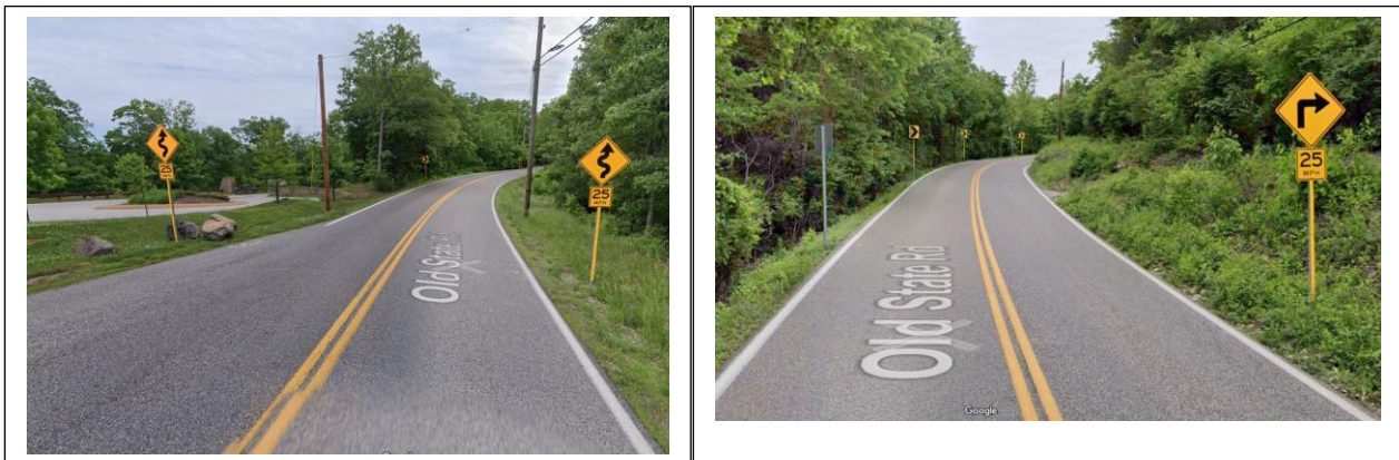
Existing Curve and Winding Road Warning Signs
